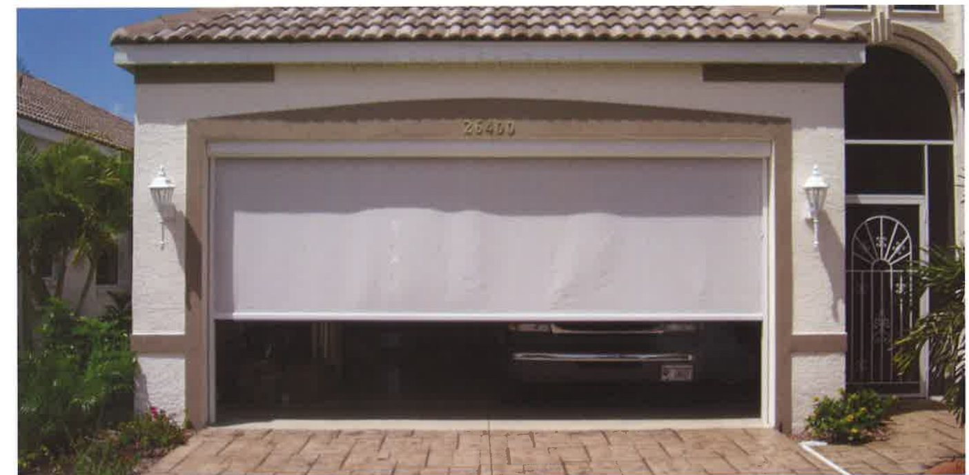
Garage room screening
